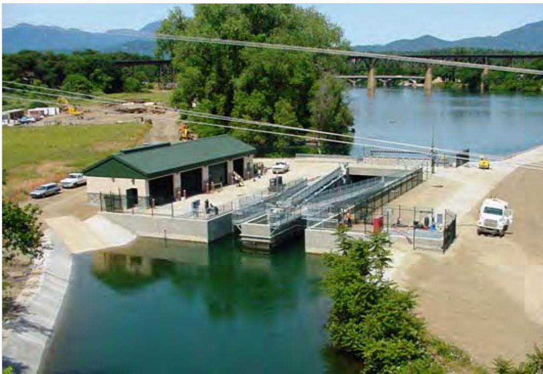
Figure 4-7. Anderson-Cottonwood Irrigation District Canal Screen
